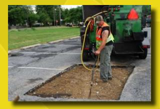
**Repairs:** Patching is simple to perform. With the flip of a switch, the operator simply discharges as little or as much hot mix as is needed.
