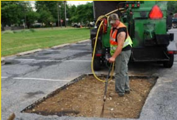
**Rake & Roll:** The PT 10-120 is easy to use and the onboard additive tank ensures quality hot mix with every batch recycled. Simplicity of use allows the crew to focus on what's most important, tack coating and proper lay down. Hot mix material is placed using standard methods. An optional plate compactor or roller can be carried onboard, completing your all-in-one mobile patching system.
