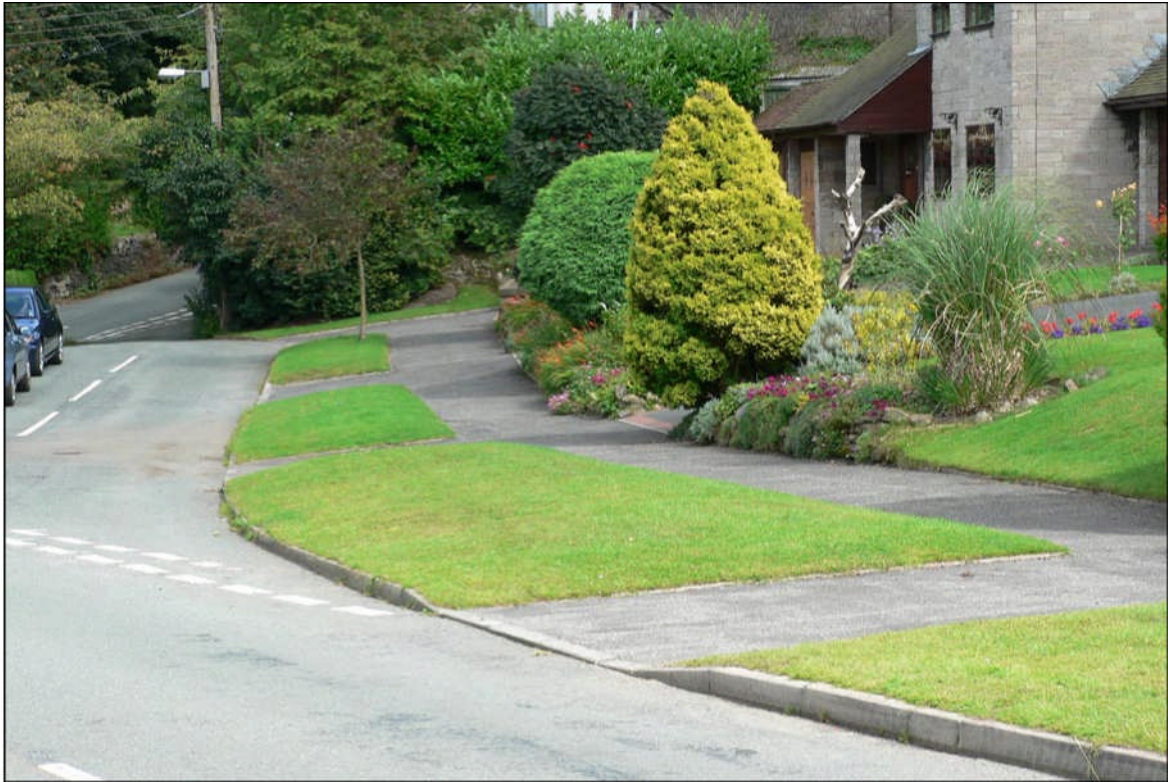
Figure 3 - The process creates minimum disruption to households, where both the footway and driveways are refurbished using the in-situ recycler
