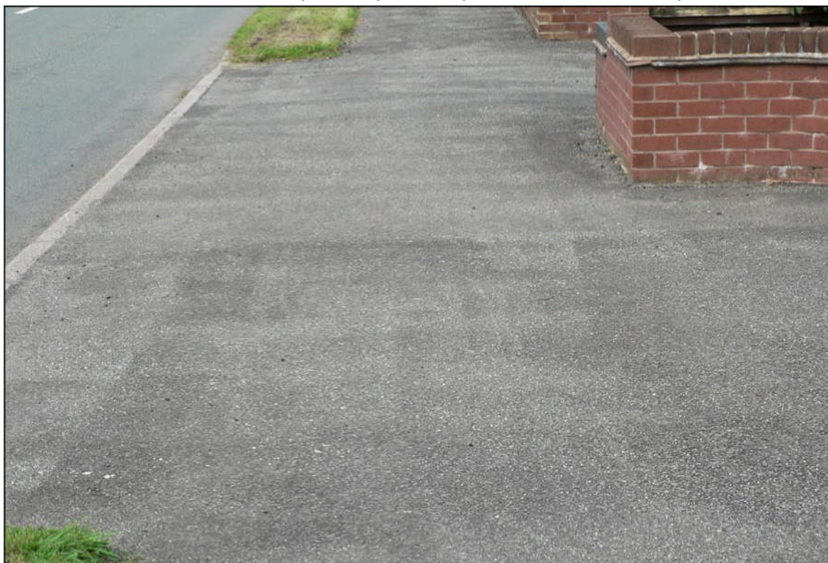
Figure 2 - A close up of the surface shows a textured finish —ideal on the steep inclines of Clewlovs Bank
