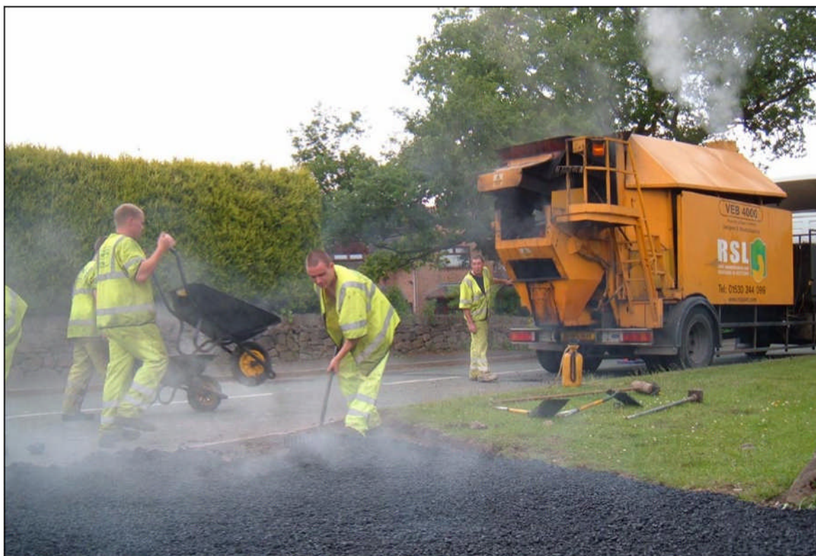
Figure 1 - A team of enthusiastic operatives take hot recycled material from the rear of the asphalt recycler to replace a worn out driveway
