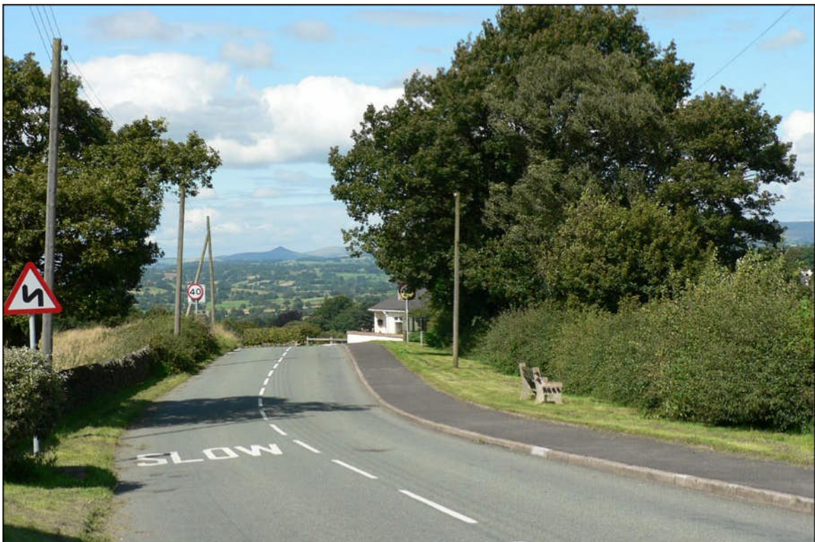
Figure 4 - The impact of replacing the footways on this steep bank with restricted working was significantly reduced by using the asphalt recycling machine
