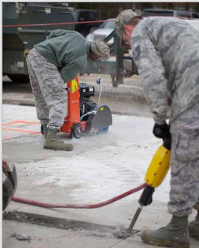
Pavements and Equipment CEs perform a variety of spall and full-depth concrete and asphalt repairs, testing equipment, tools, and materials included in the SuPR Kit. (photo by Mr. Eddie Green)
